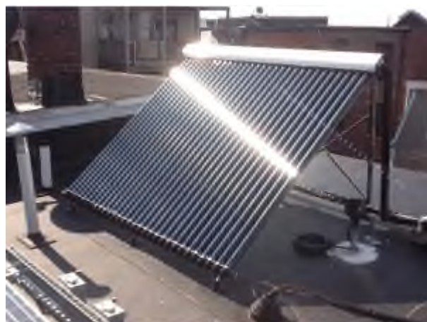
Residential Evacuated Tube System - Boston, MA
