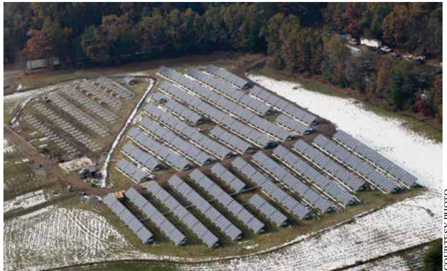
Easthampton's 2-megawatt solar array, which went live on June 8, is one of the largest ground-mounted solar projects on a landfill in the state.
