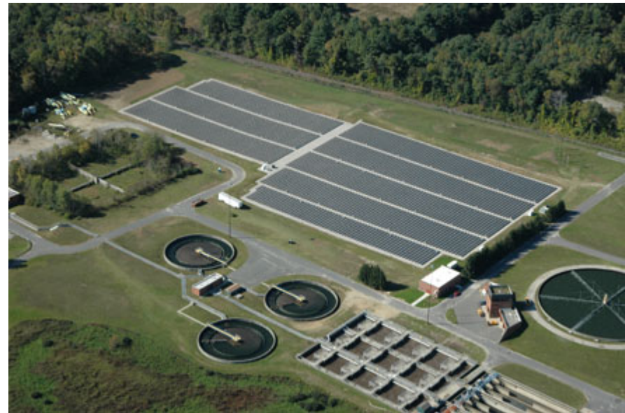
1.6 MW PV System at Pittsfield WWTP
