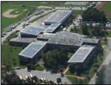
Mashpee High School 300 kW
