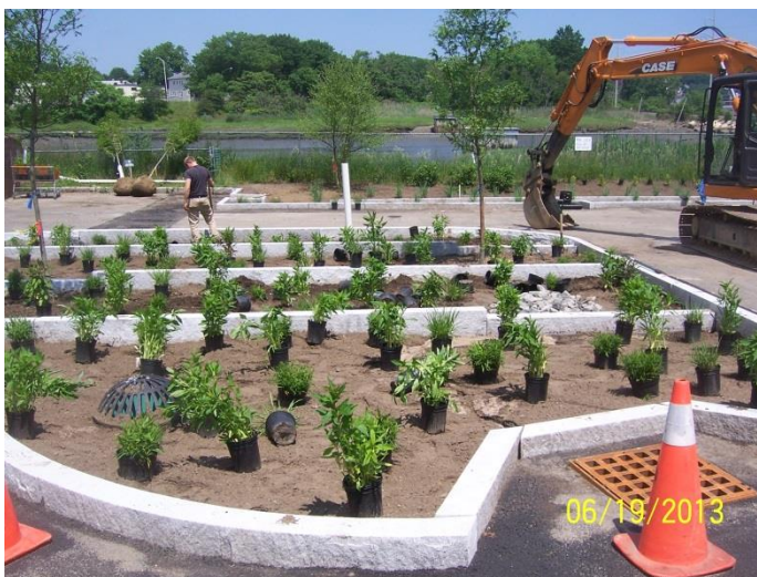
Figure 1 - Rain gardens, such as this installation at the Mace Public Housing Project in Chelsea, help to reduce flooding and water pollution by collecting, storing, and naturally filtering stormwater runoff before it enters sewer systems. Source: City of Chelsea Dept. of Public Works
