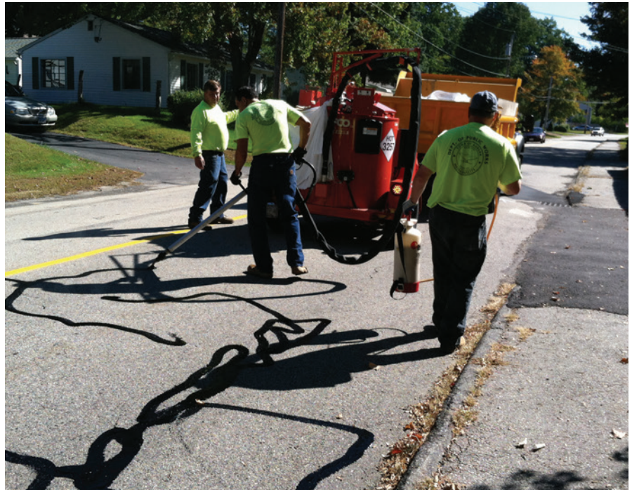
Auburn has an aggressive crack-sealing program to extend the life of its roads. (Courtesy photo)
