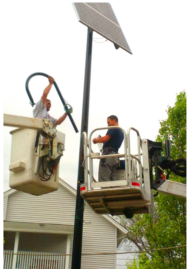
Workers install networked, grid-connected and off-grid (solar and battery) “smart” lighting with sensing along a community bike path in Somerville.
