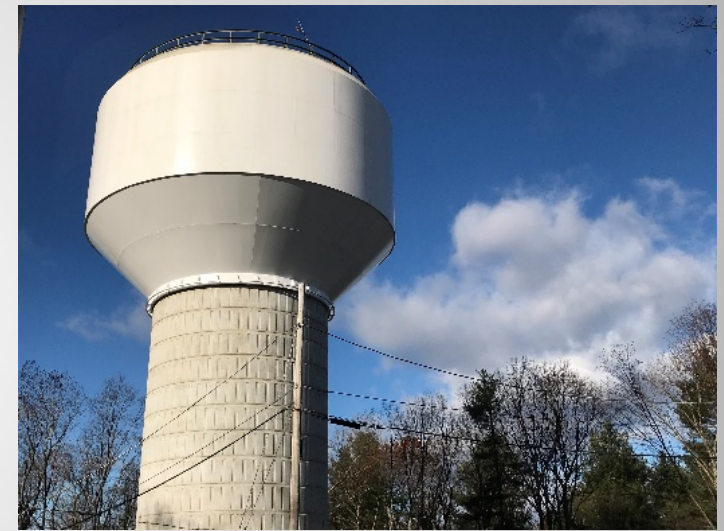
Prospect Hill Water Tank
