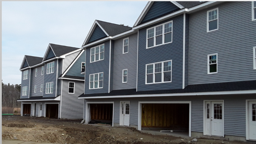
110 Place - 19 Littleton Road
