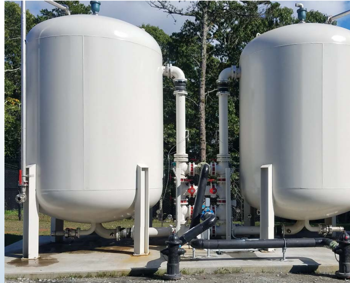
PFAS Removal Pressure Vessel Installation (Hyannis, Massachusetts)
