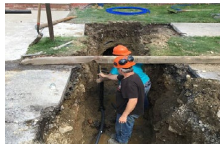
Malden is using American Rescue Plan Act funds to speed up the removal of lead pipe service lines and has developed a new tool to identify lines in areas that serve children. (Photo courtesy city of Malden)
