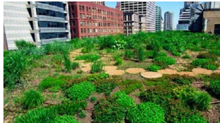
Climate-friendly green roofs, like this one at Chicago's City Hall, can reduce building cooling costs while also absorbing rainfall. (Photo courtesy National Park Service and city of Chicago)
