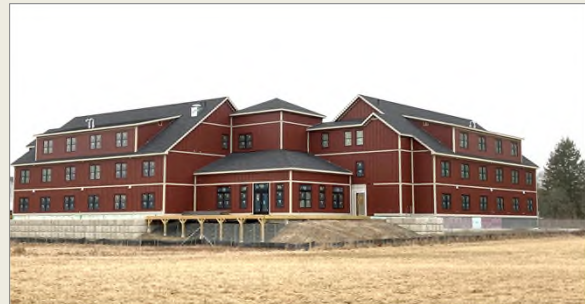
Sanderson Place Senior Housing Development, Sunderland
