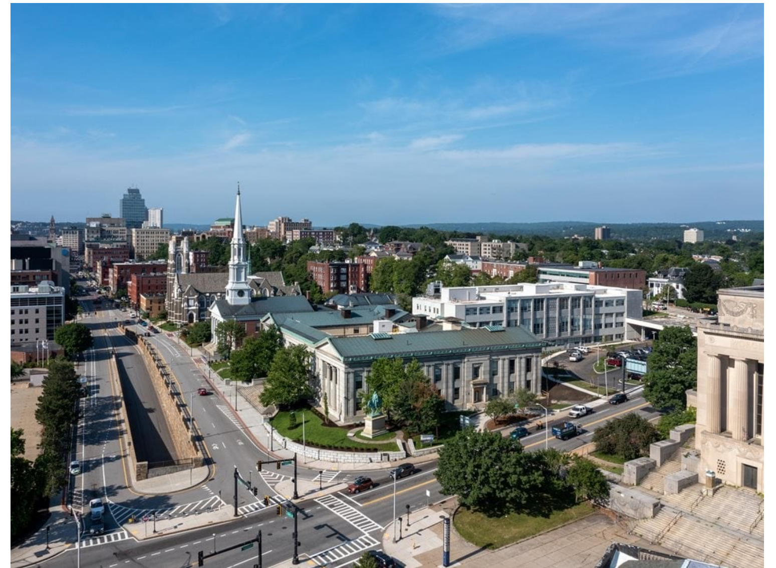
Courthouse Lofts, Worcester Former Court Building
