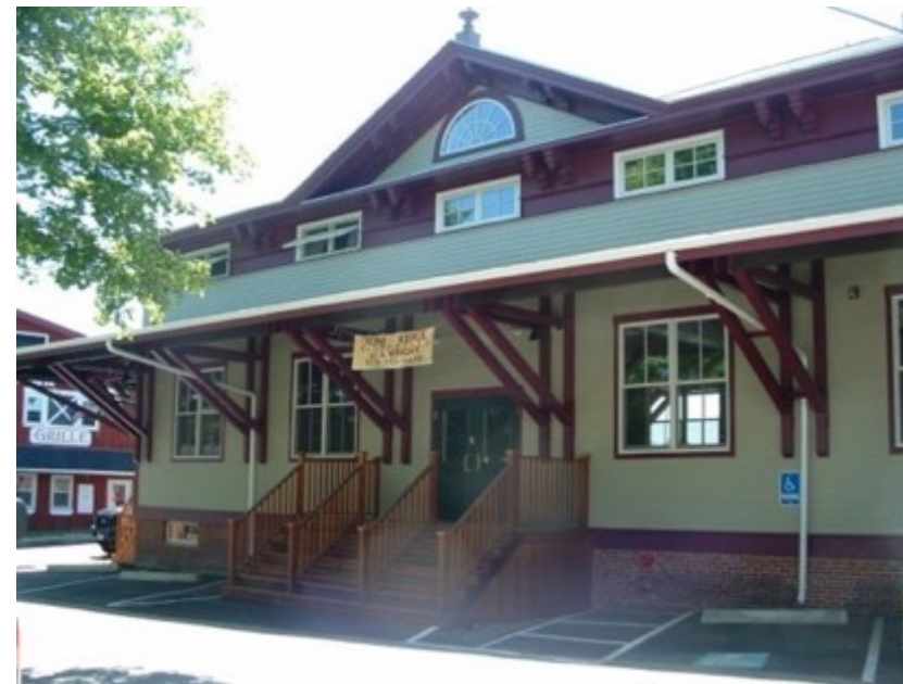
Elm Street Amesbury Former Train Depot
