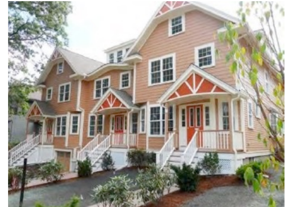
Oakley Neighborhood, Belmont Former Church
