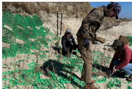
Nantucket town staff install cliff stabilizers on Madaket Beach as part of a pilot program to reduce erosion. (Photo courtesy town of Nantucket)
