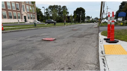
A bond bill passed by the House on April 15 would authorize $300 million for the Chapter 90 local road and bridge program for fiscal 2027.
