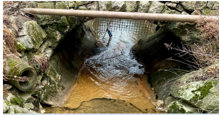
Culverts are among the climate resiliency projects being funded by $45 million in grants awarded through the new Environment and Climate One Stop program.
