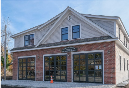
The post-renovation Bank Street Firehouse has three one-bedroom apartments, an office space, and a community gathering space. (Photo courtesy Harwich Conservation Trusts/Gerry Beetham)
