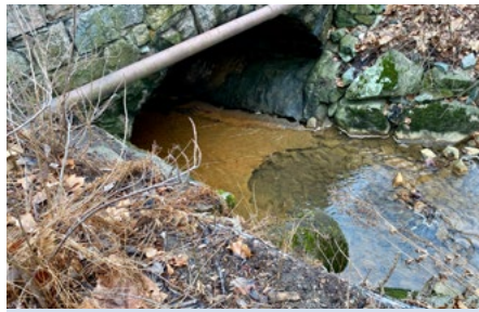
The Massachusetts Division of Ecological Restoration recently announced a total of $750,000 in awards to seven communities for culvert replacement assistance.
